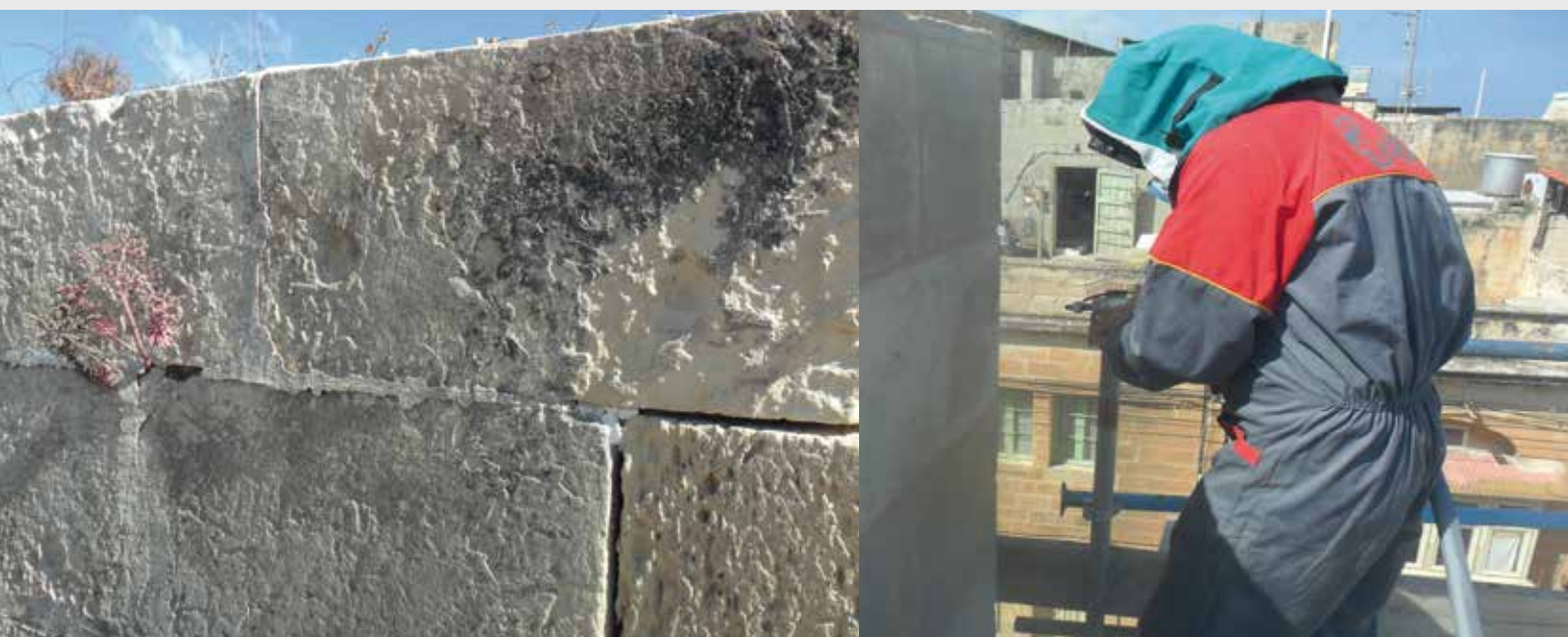
Restoration, removal of black crusts and salt efflorescences with HELIX® air-abrasion technology
