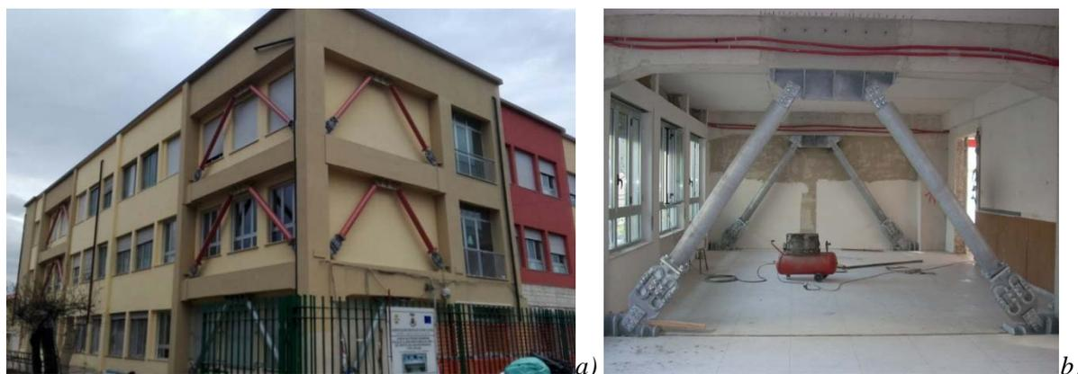
Figure 8: The building after retrofit: a) External view. b) Detail of braces fitted with hysteretic dampers.
