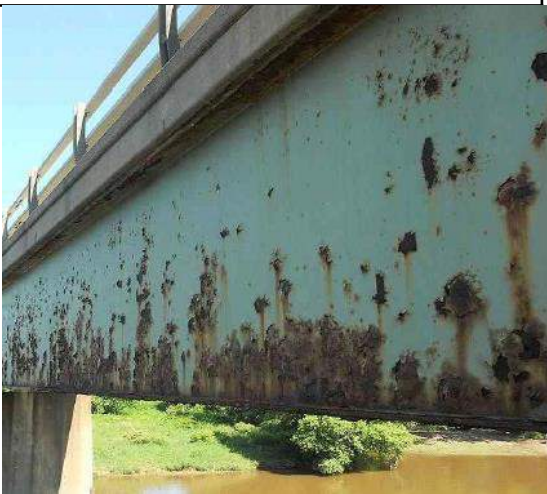
Fonte: BRIDGE INSPECTION MANUAL – NY’S DOT
