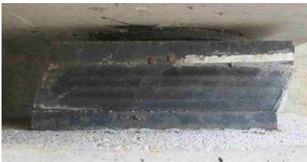
Fonte: BRIDGE INSPECTION MANUAL – NY’S DOT
