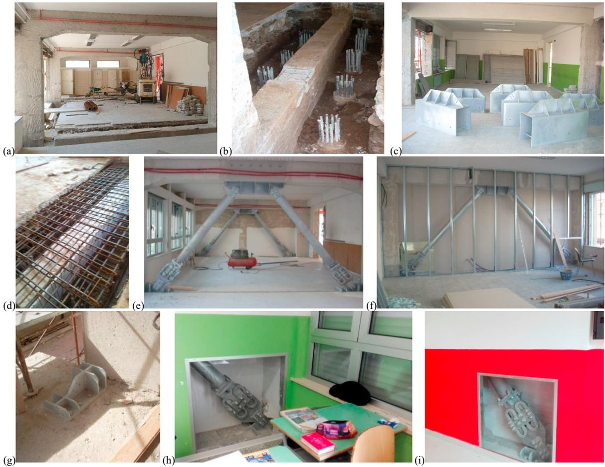
Fig. 6. (a) Excavations in foundation; (b) Construction of micropiles; (c) Connecting plates of damped brace to beam; (d) Rebars in foundation slab; (e) Internal damped braces; (f) Construction of partitions; (g) Connection of damped brace to foundation; (h) - (i) Visible dampers.
